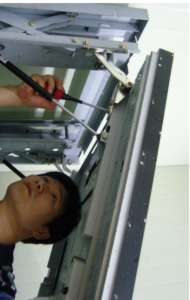
9. Fixing the bracket and panel with M5 screws (12 points)
